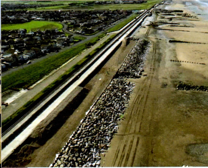
Completed section of lower rock revetment looking south.
